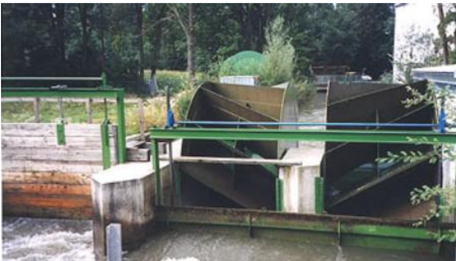
Fig. 6: Pilot Plant, upstream view
